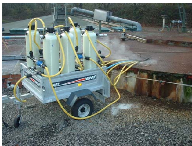
Figure 17. The pilot rig employed at the Stubbins Mill site
