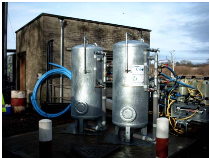
Figure 10. The two full-scale filters at Malton WwTw, one packed with sand medium the other with medium grade glass
